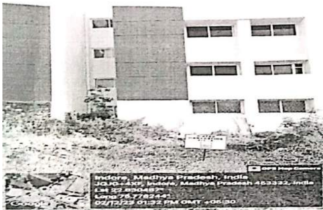
Rain water harvesting system: 01
