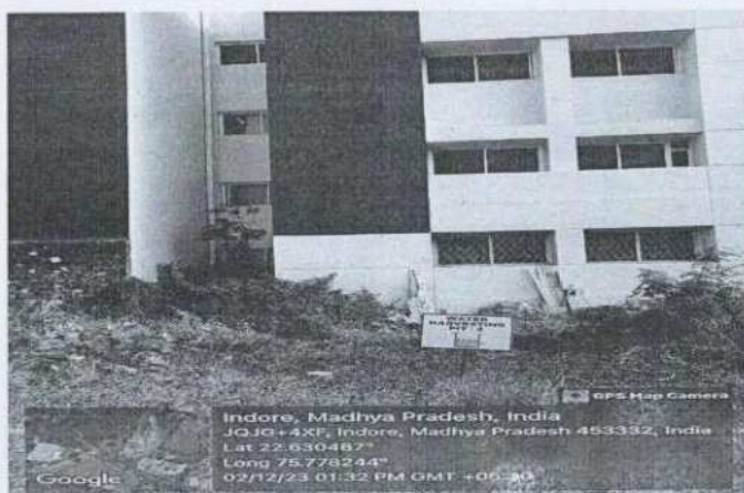
Rain water harvesting system: 01
