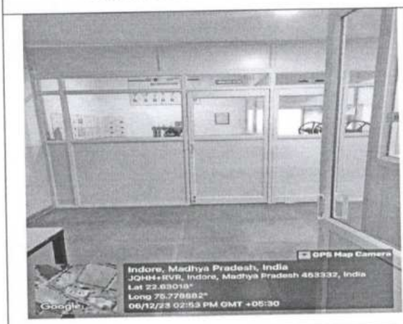
Machine room: Front view
