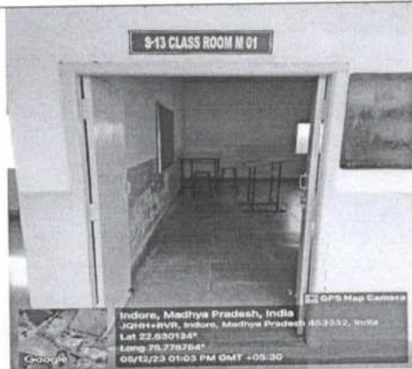
Classroom M1: Front view
